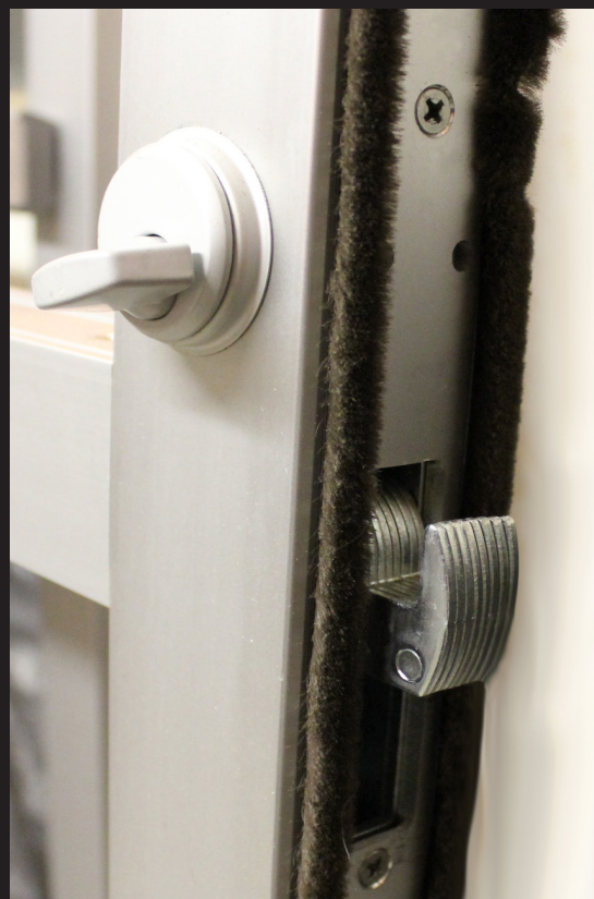
Armored Strike Retrofit
